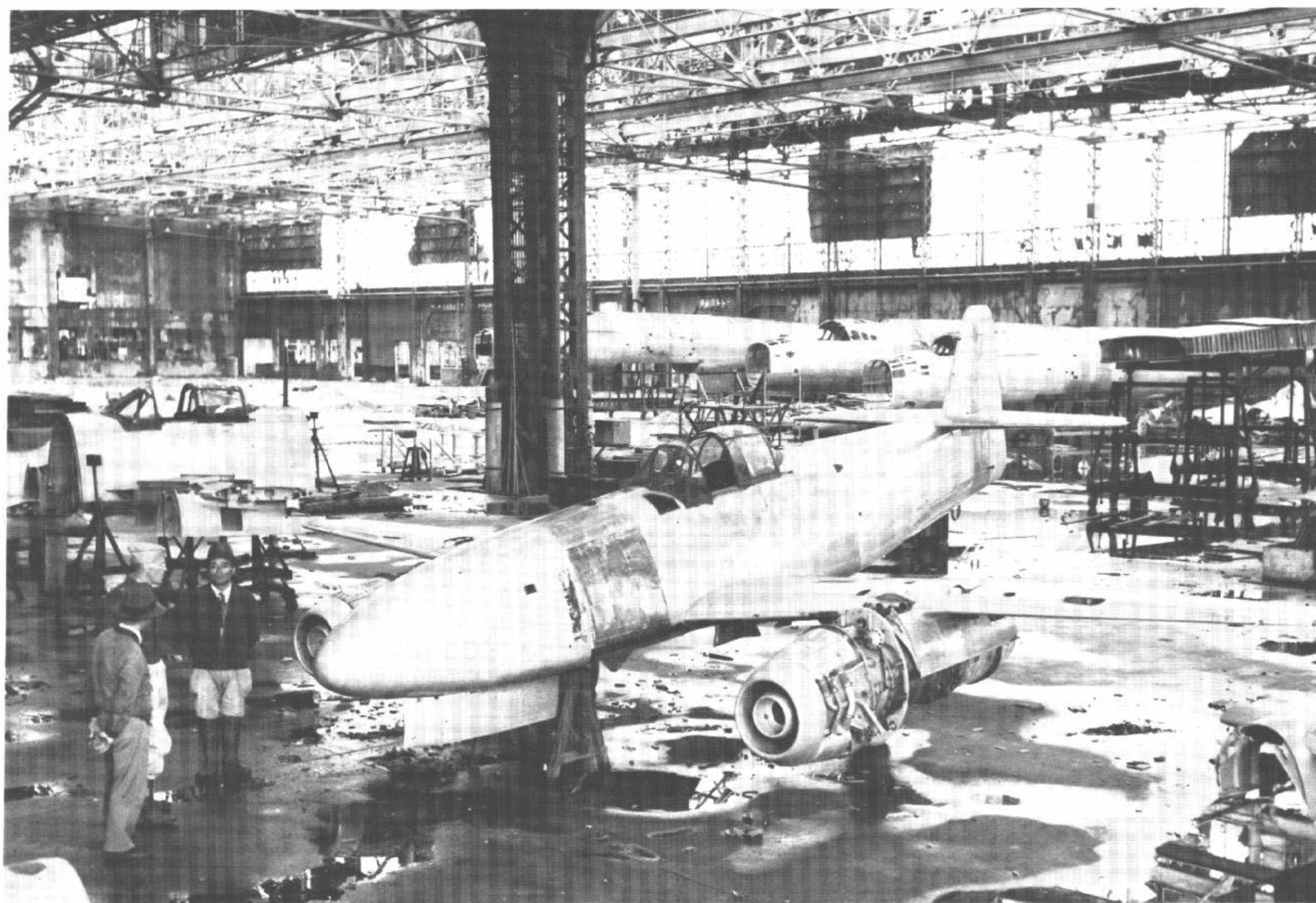
This view of the final assembly line of Kikka was taken on November 6, 1945, at Nakajima's Koizumi plant, nearly three months after the war. In the background are three fuselages and wing sections of unfinished 4-engine Renzan Navy bombers. Production on these aircraft terminated so that efforts and material could be concentrated on Kikka.
