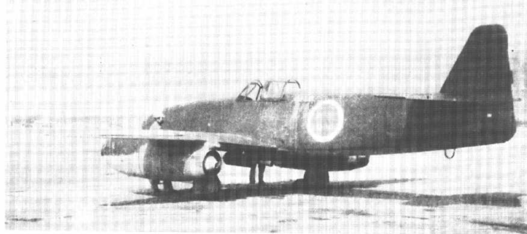
RATO tubes are in place under the wing of Kikka for its second flight. The stabilizer sat high on the fuselage, well away from the jet exhaust. Flight control surfaces were fabric and dope covered, an unusual arrangement for tail surfaces exposed to varying degrees of heat during engine ground operations.
